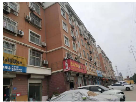
图2-6 110kV涓南线#40-#41线南21m永康佳苑居民楼
