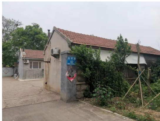
图2-11 110kV涓南线#45-#47线南3m看 护房
