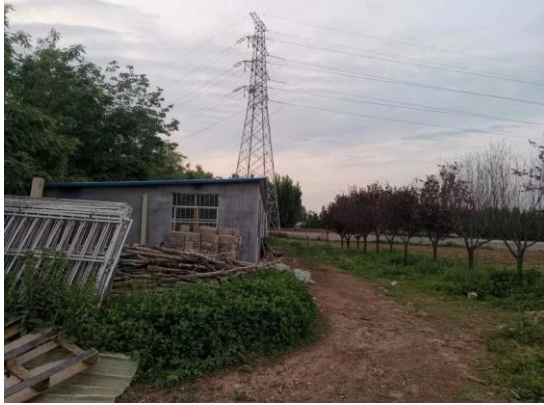
图2-19 110kV涓王线3#-2#线东10m看护房
