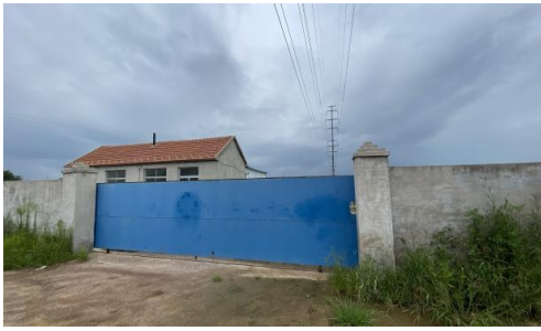
图2-9 110kV 镆赵线68#~69#塔间线下空心砖作坊
